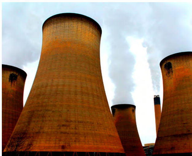
Figure 10.24 Cooling towers at the Drax power station in North Yorkshire, United Kingdom (credit: Les Haines, Flickr)
